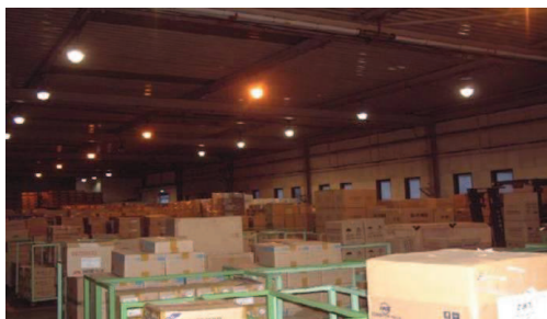
Before: 175W HPS and 150W Metal Halide
