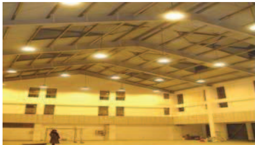
Before: 400W High Pressure Sodium
