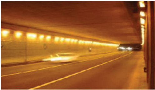
Before: 250W High Pressure Sodium
